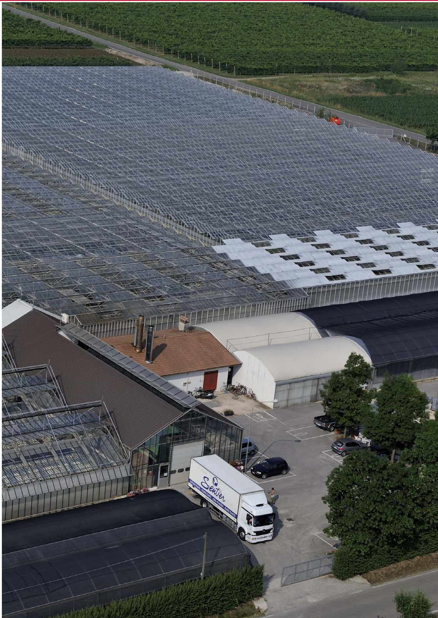
PANORAMICA AZIENDA SENTIER - VIEW OF COMPANY SENTIER
